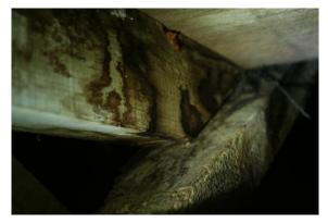
Rainwater ingress noted to roof void over Bedroom 6. Valley issues and also rear hip rafters were wet. Check hips externally and valley gutter.
