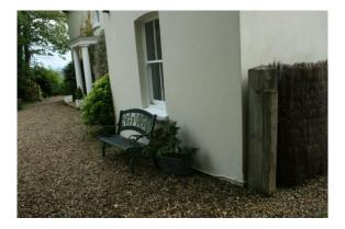
(iv) Cracking was noted in the render to the side (northwest) elevation. Rake out and renew. These cracks are historic and are not structural in our view.
