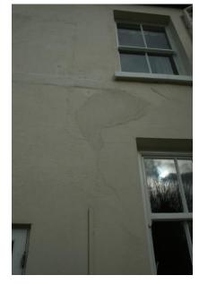
(vi) Cracking was also noted to the rear (southwest) elevation around the En-Suite projection from Bedroom 1.
