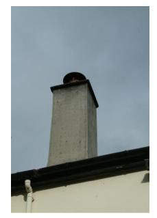
There is a stainless steel flue, also to the same elevation, which takes the flue from the oil fired boiler located in the boiler room. Also sound. No sign of any defects.
